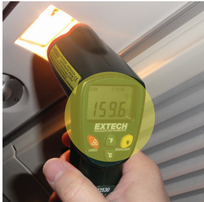
Temperature reading of incandescent bulb at about 160 deg F. - It is quite a bit warmer!
